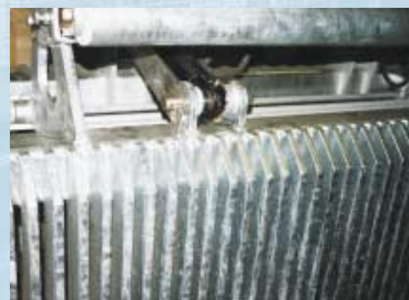
For river intakes the grab is galvanised, it can however be constructed in bronze or stainless steel.
